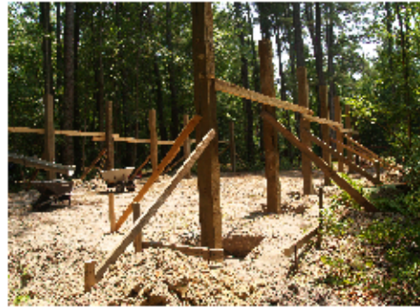
New 24' x 48' Multi-purpose Activity Pavilion Under Construction
